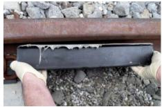
Press the opposite component (**STRAILastic\_A** fixing paste applied here as well) as parallel as possible onto the rail and mount the other half of the fixing clamp onto the fixing pins.
