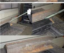
Remove the **STRAILastic\_A** rail damper from the rail using a crowbar or something similar (avoid damaging the damper).
