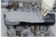
Press the rail damper with applied **STRAILastic\_A** fixing paste onto the rail (install as much as possible in the middle of the sleeper bay) and pass the part of the fixing clamp with the fixing pins under the rail.
