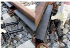
After the rail dampers with applied **STRAILastic\_A** fixing paste have been properly positioned on both sides of the rail and assembled using the **STRAILastic\_A** fastening kit, fix as follows:
