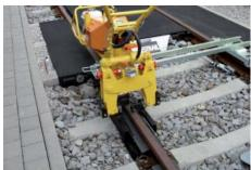
Using the **ROBEL Fast-Clip-Machine** (incl. special attachable **STRAILastic\_A** attachment) the clamps are pressed into the sleeper bay, so that the clamps snap into their final position.
