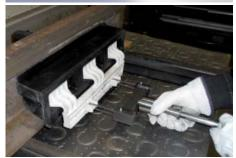
Shove the slide hammer handle removal aid **STRAILastic\_A** with some force in direction of the **STRAILastic\_A** fixing clamp.
