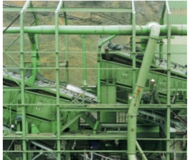
Installation performed by HAYER specialists
