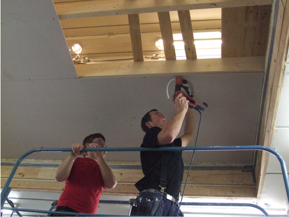
Figure 8 – Mounting of the ceiling consisting of two layers of 13 mm gypsum boards.
