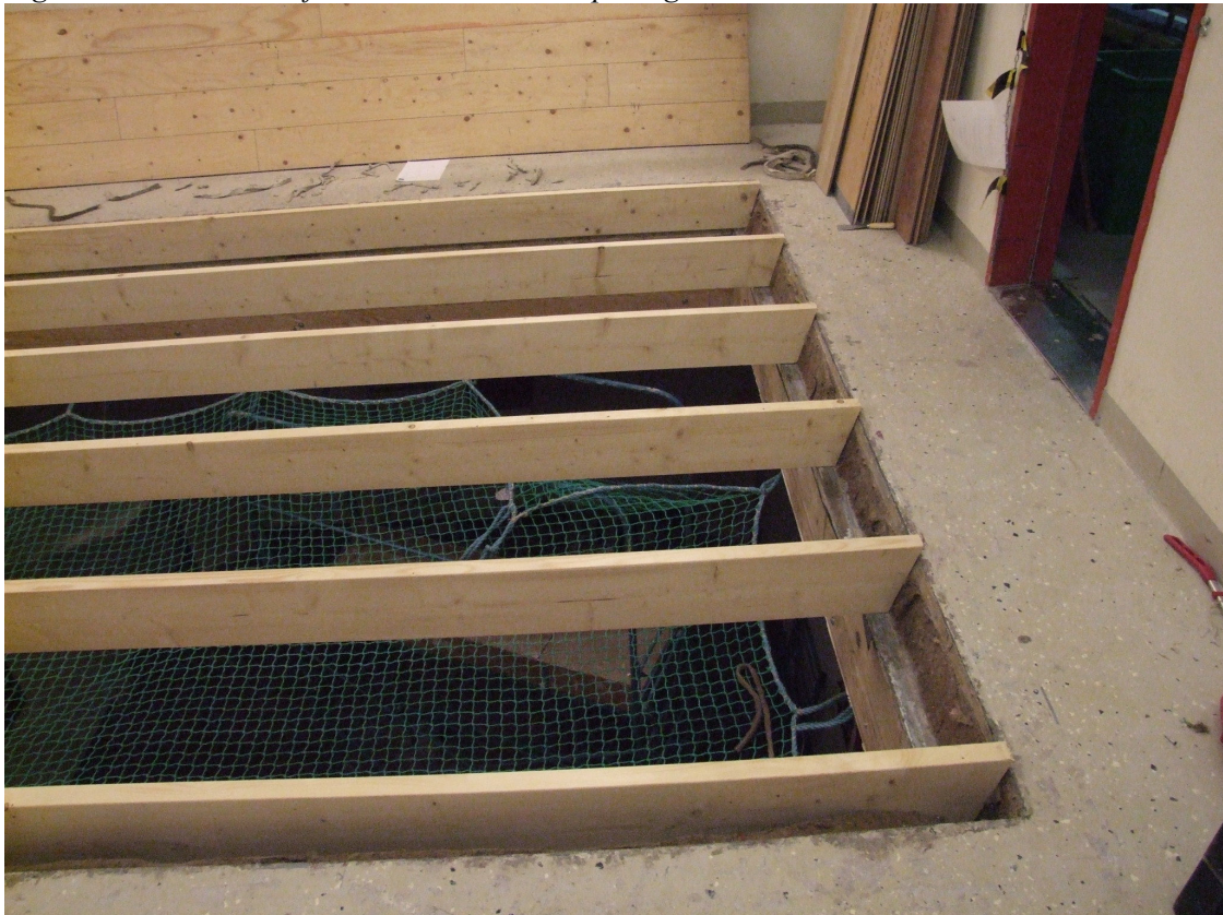
Figure 7 – Placement of the studs in the test opening.
