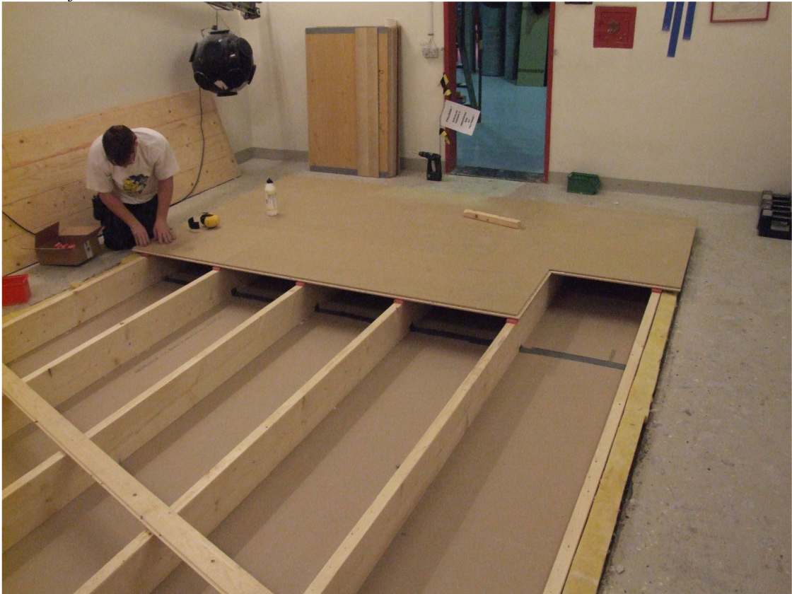
Figure 14 - Building of upper floor called P12 (with p12 sylomer) on the clean version of the wooden floor structure.
