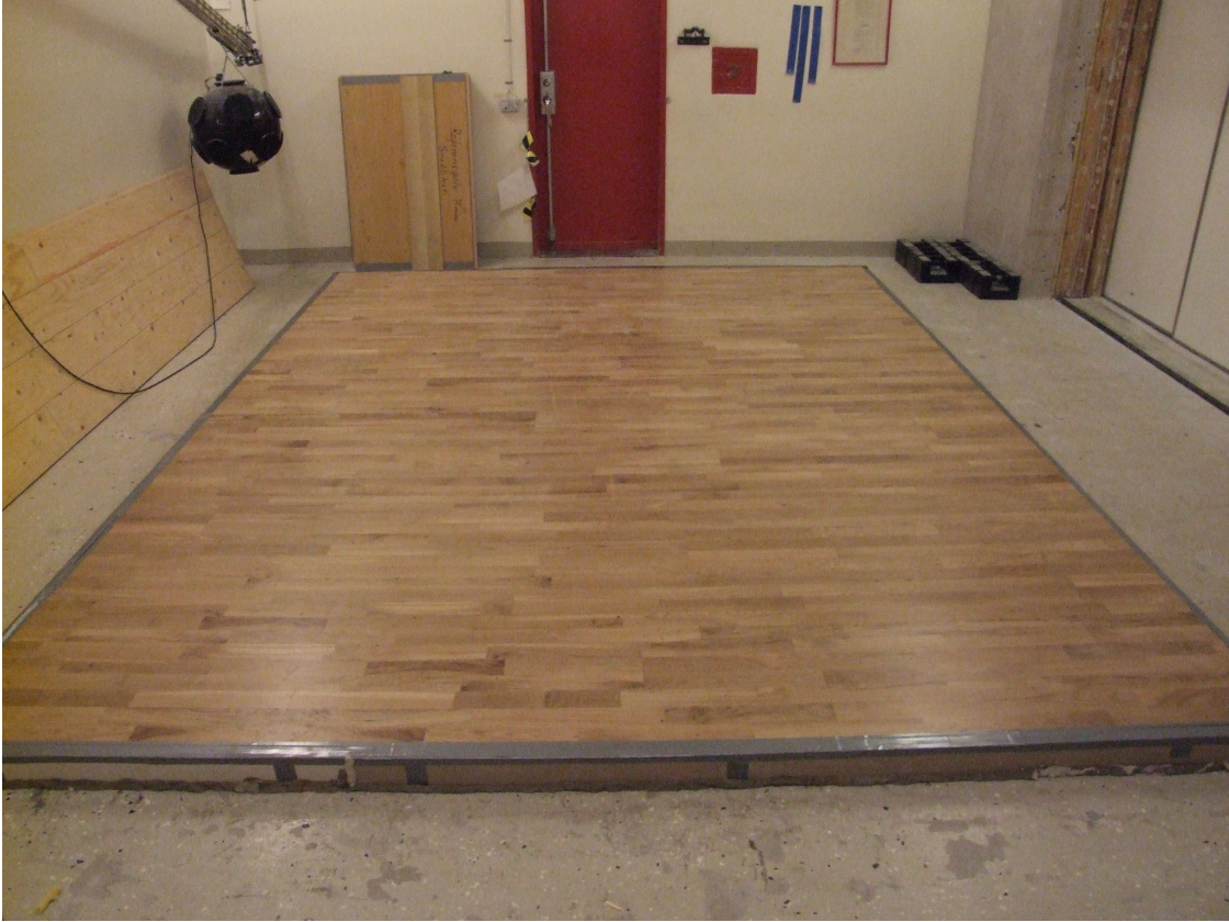
Figure 18 – Parquet floor finished..
