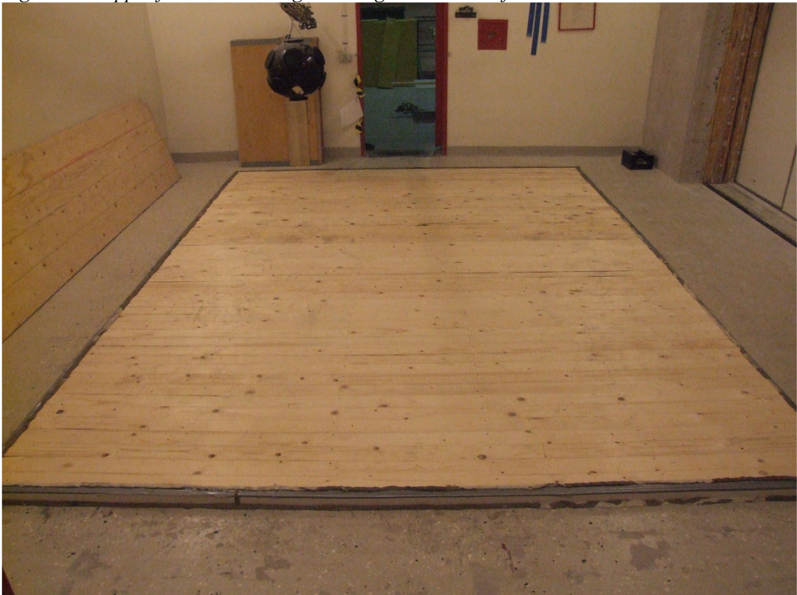
Figure 11 –Upper floor 22 mm tongued and grooved board finished.
