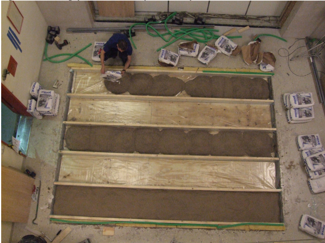
Figure 20 – Building of the sand version of the wooden floor structure.
