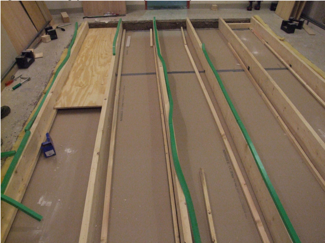
Figure 19 – Building of the sand version of the wooden floor structure.
