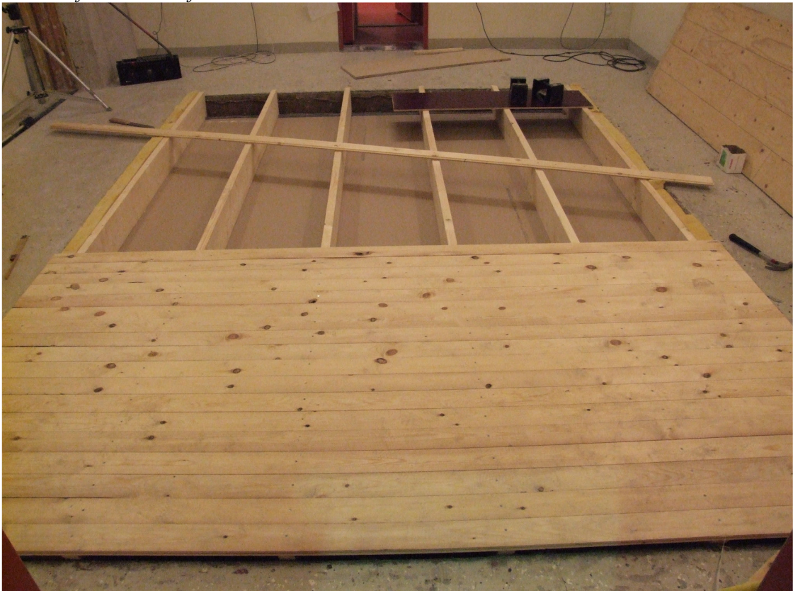
Figure 9 - Building of the first upper floor (22 mm tongued and grooved board) on the empty version of the wooden floor structure.
