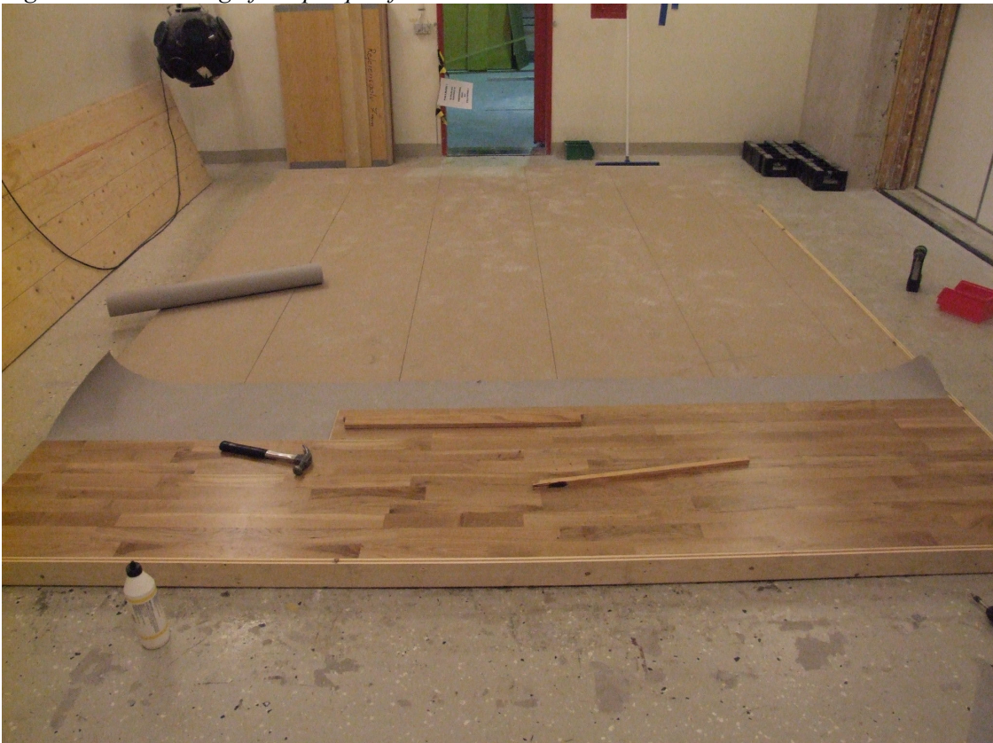
Figure 17 – Mounting of the parquet floor.
