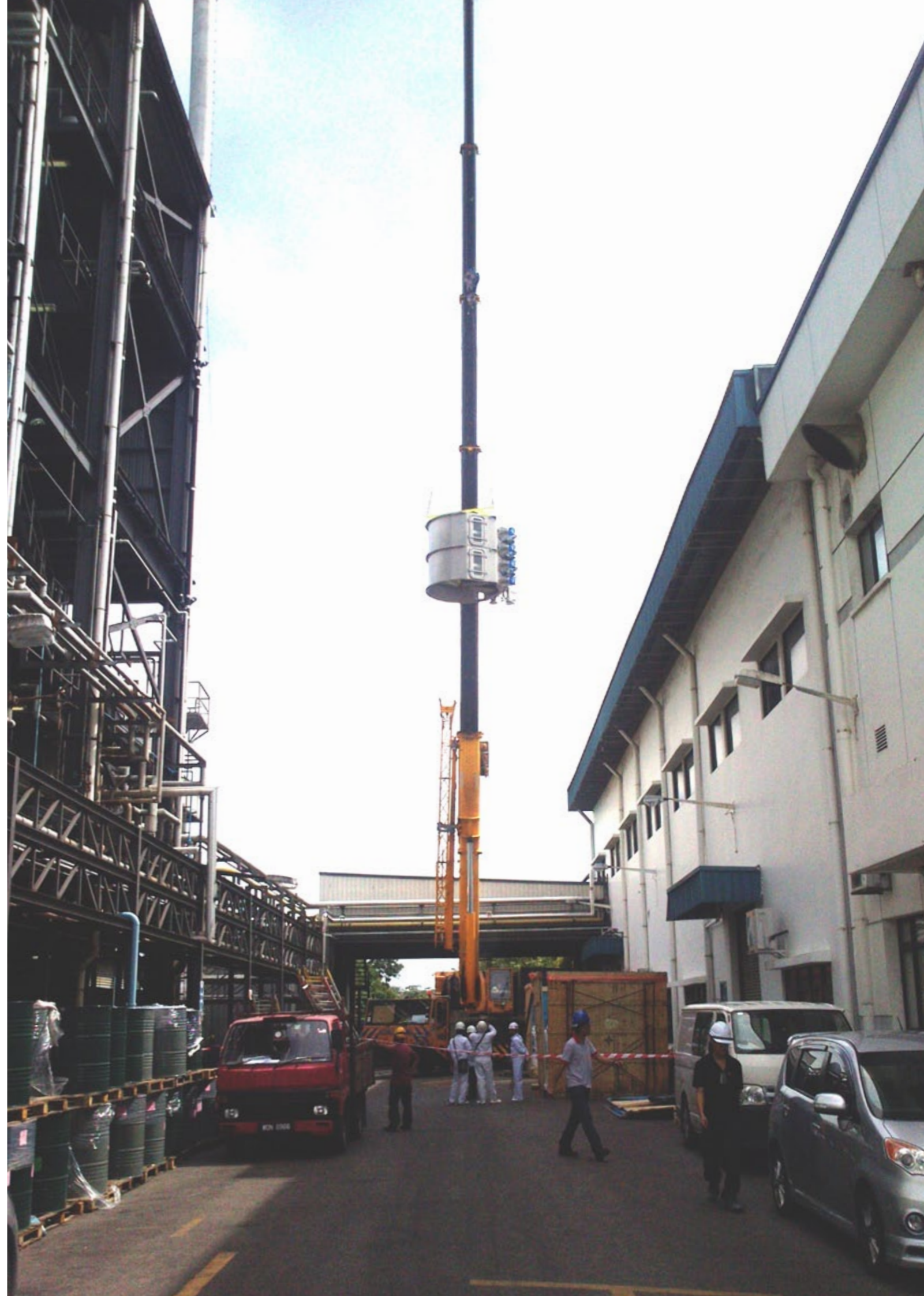
Installing a disc pastillator ▶
